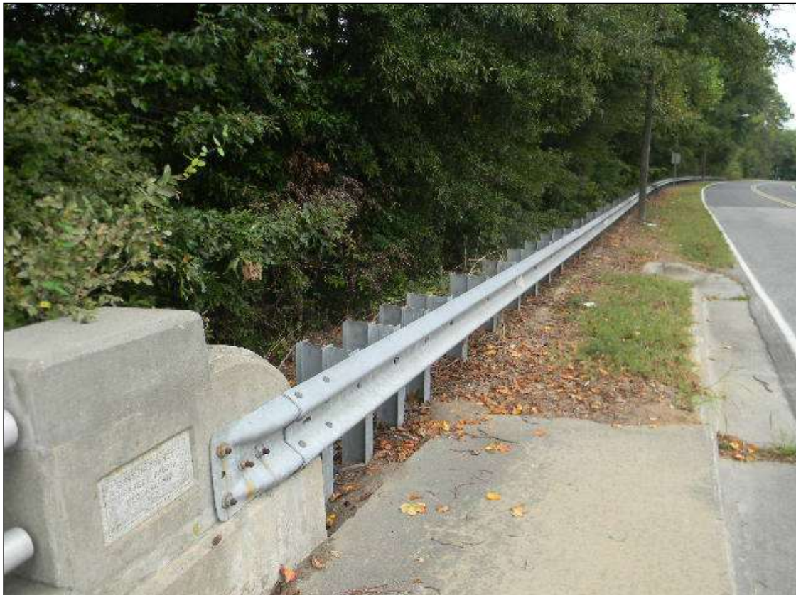
TYPICAL GUARDRAIL CONNECTION AND POST SPACING. SW CORNER SHOWN.
