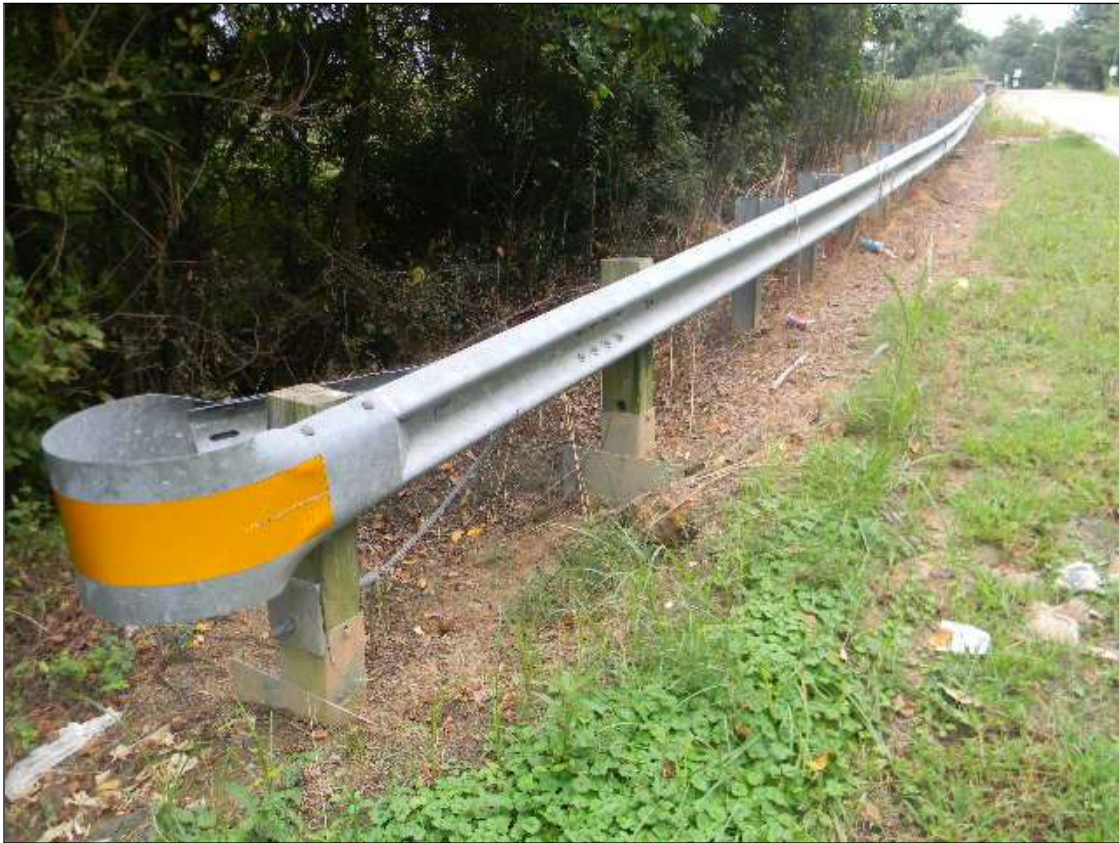
TYPICAL GUARDRAIL END AND POST SPACING. NW END SHOWN.
