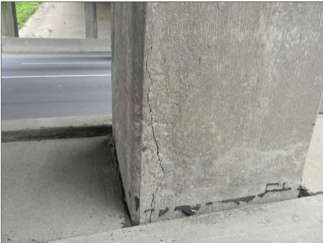
VERTICAL CRACKING WITH IMMINENT CORNER SPALLS ARE PRESENT ON COLUMNS 1 AND 3 AT BENT 2.
