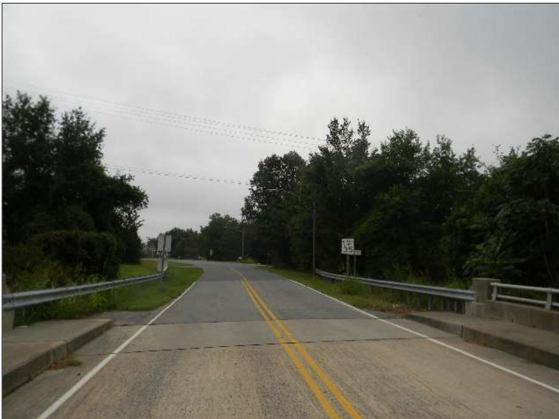
GUARDRAIL LOOKING EAST
