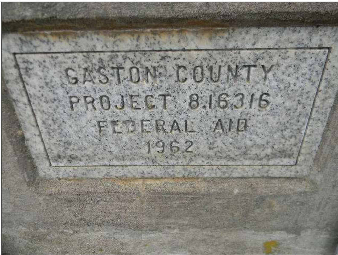
BRIDGE INFO PLATES AT THE SW AND NE CORNERS.
