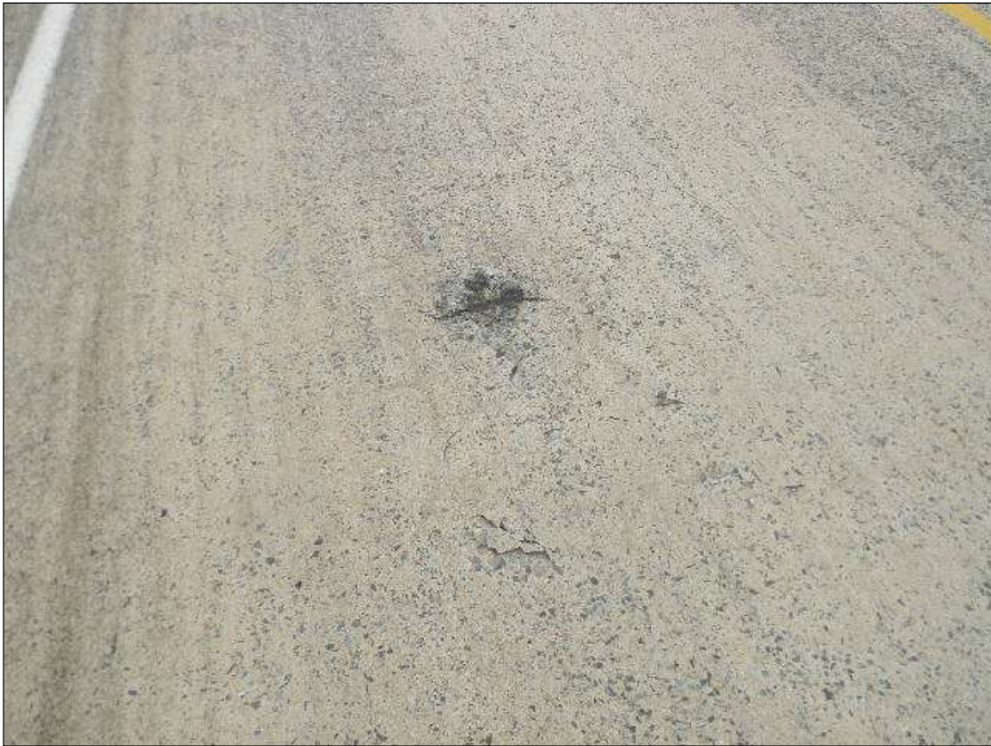
SPAN 4 ROADWAY SURFACE HAS A 6 INCH LONG BY 6 INCH WIDE BY 1/2 INCH DEEP SPALL WITH EXPOSED REINFORCEMENT IN THE WESTBOUND LANE. SPAN 1 HAS A SIMILAR
