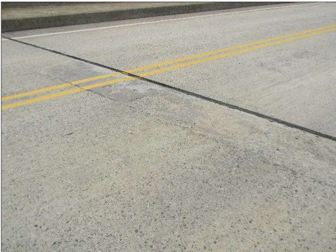
SPAN 1 DECK ROADWAY SURFACE HAS A 2 FT LONG X 12 FT WIDE AREA PATCHED ALONG BENT 1 JOINT WITH BREAKING UP OF THE PATCH IN THE EASTBOUND LANE.
