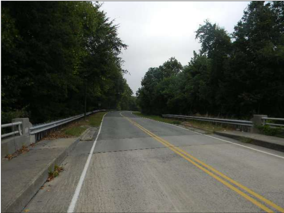
GUARDRAIL LOOKING WEST
