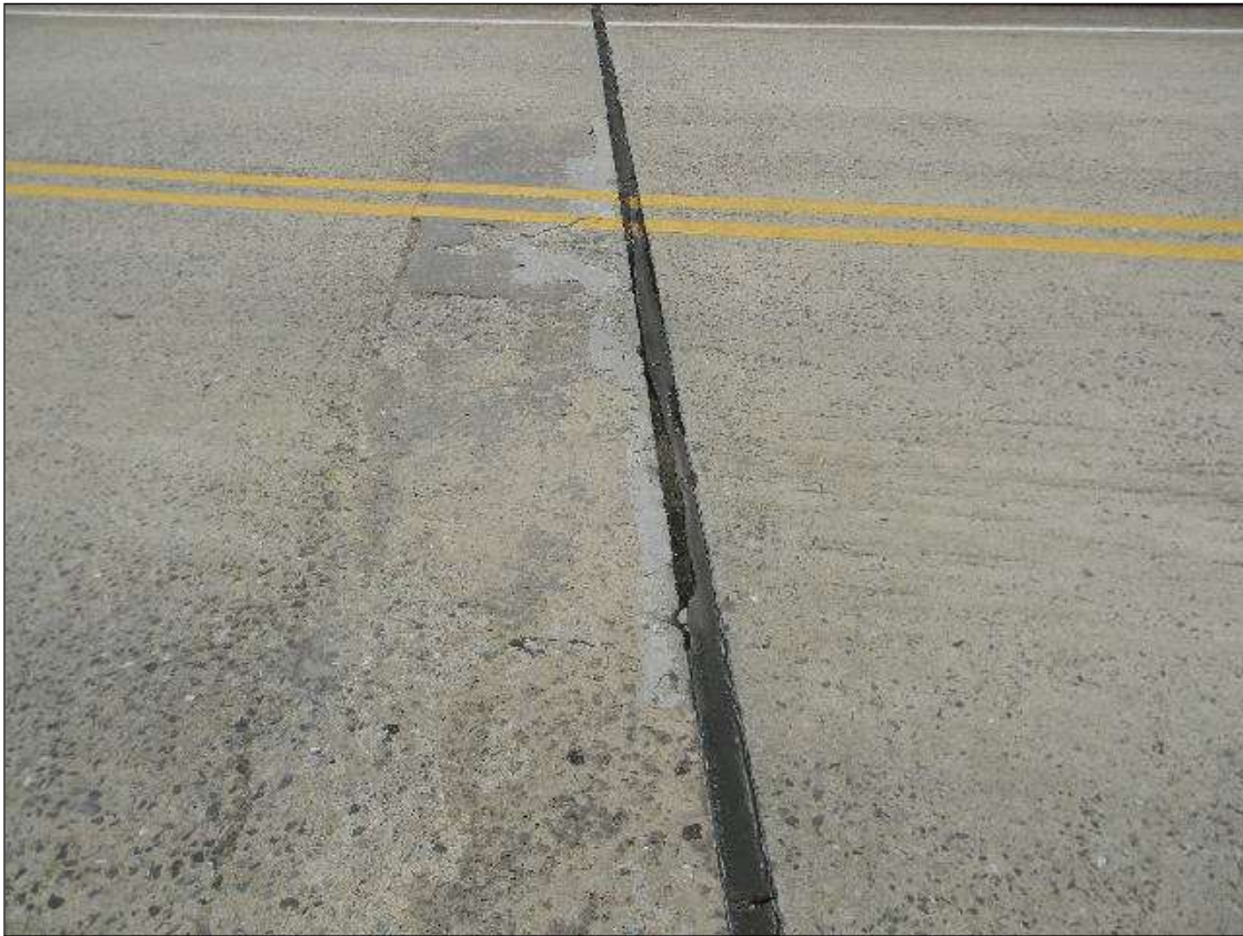
JOINT SEALS AT BENTS 1 & 3 AND ABUTMENT 2 HAVE SETTLED 1/2 INCH AND ARE ALLOWING SAND ACCUMULATION IN THE JOINTS.
