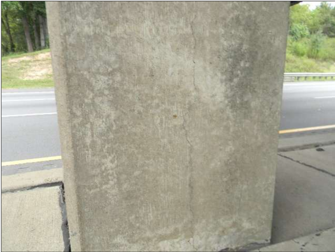
BENT 2, COLUMN 1 EAST FACE HAS A 4' LONG VERTICAL H/L CRACK IN THE CENTER. THERE ARE SEVERAL COLUMN FACES WITH THESE CRACKS.
