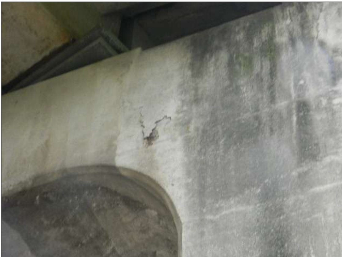
EAST FACE OF BENT 3 CAP HAS A 1' DIAMETER SPALL UNDER BAY 1.
