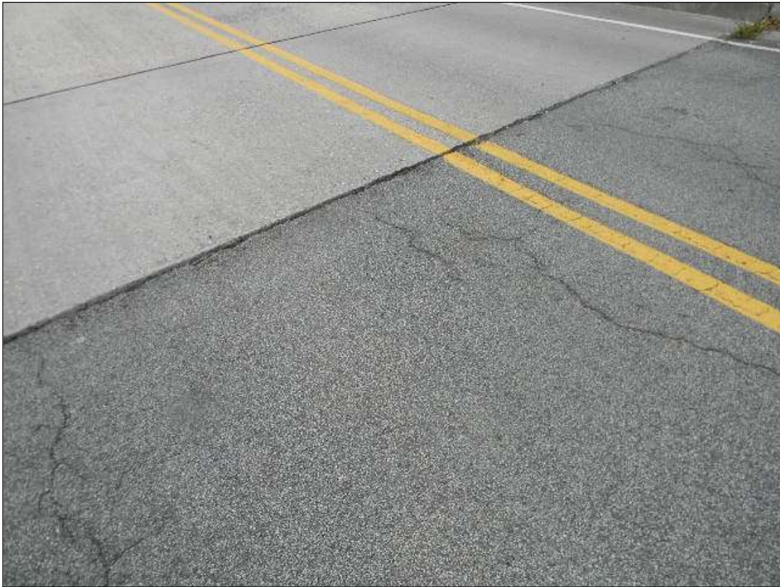
THE APPROACH ROADWAYS ARE CRACKED AND SETTLED 1/2" ALONG THE FILLFACES.
